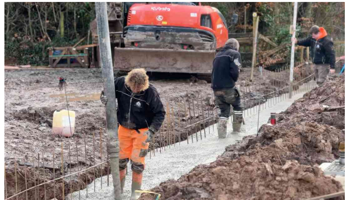
Steel reinforcement, and pumping concrete
