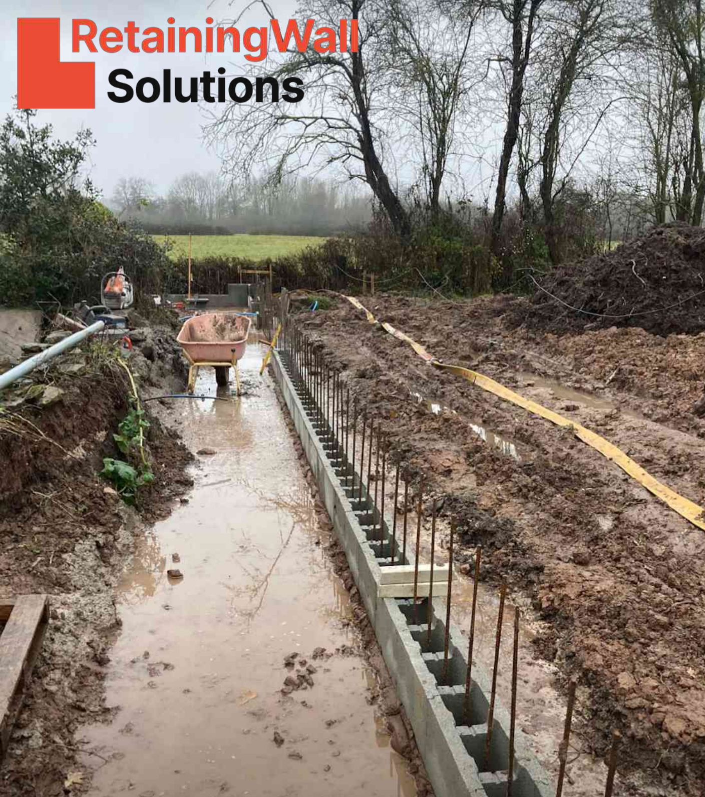
Laying the first layer of blocks
