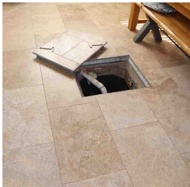
Three submersible sump pumps installed in chambers below the floors, all are interlinked with pipework.
