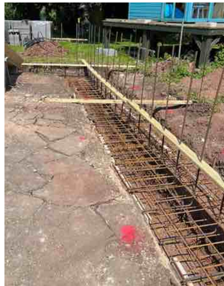
We used timbers with holes drilled, to ensure the bars remained correctly spaced and vertical during the pour
