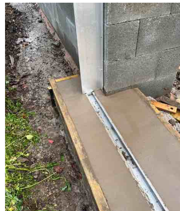
The lower part of these brackets would be embedded in the sand/cement mix that made-up the sill of the opening.
