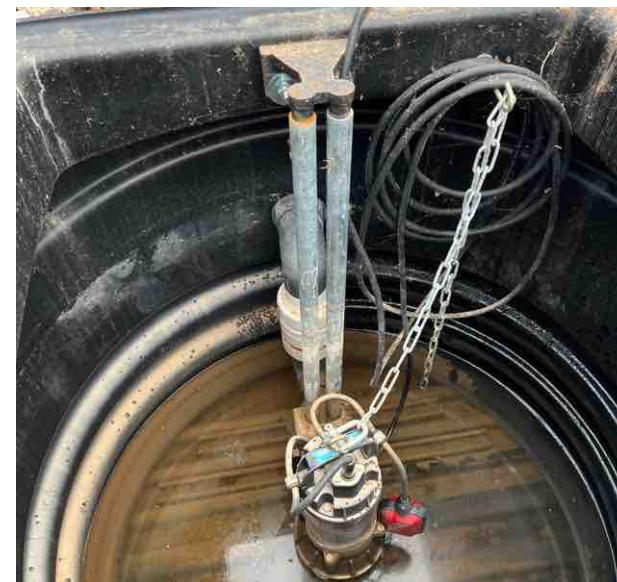
The sump has a rail system for easy replacement of a failed pump
