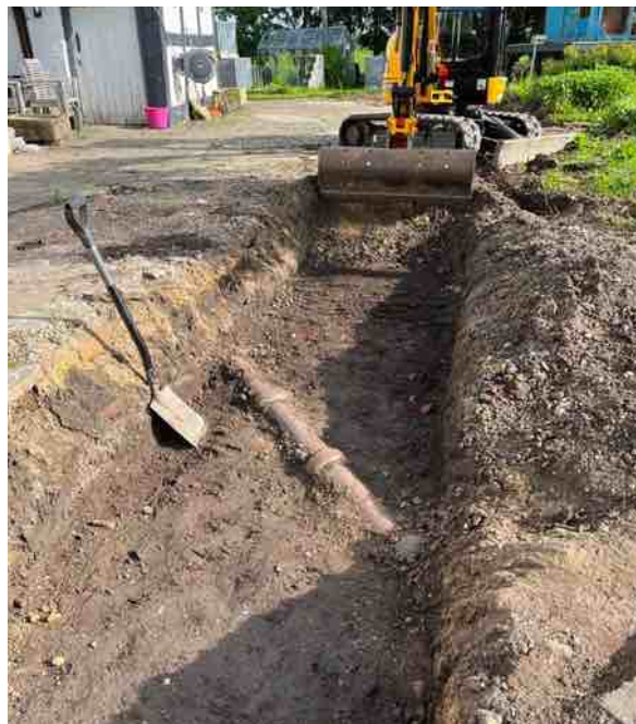
Initial foundation dig
