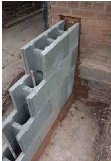
Where the wall joined the garage block it was cut into the existing brickwork to ensure stability and a strong watertight seal.
