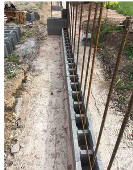
The pre-cut lengths of bars were placed in the groove in the block and tied to the vertical rebar
