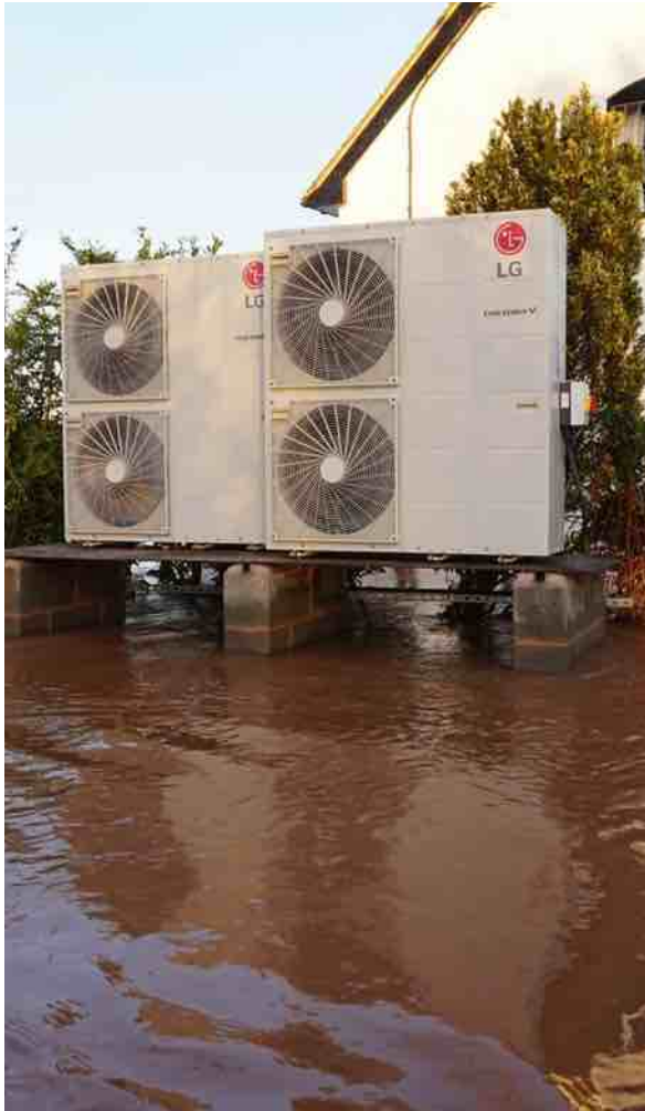
Air source heat pumps have been placed up away from flood risk.
