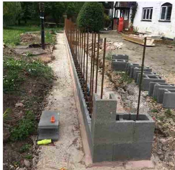
Second and third courses dry laid
