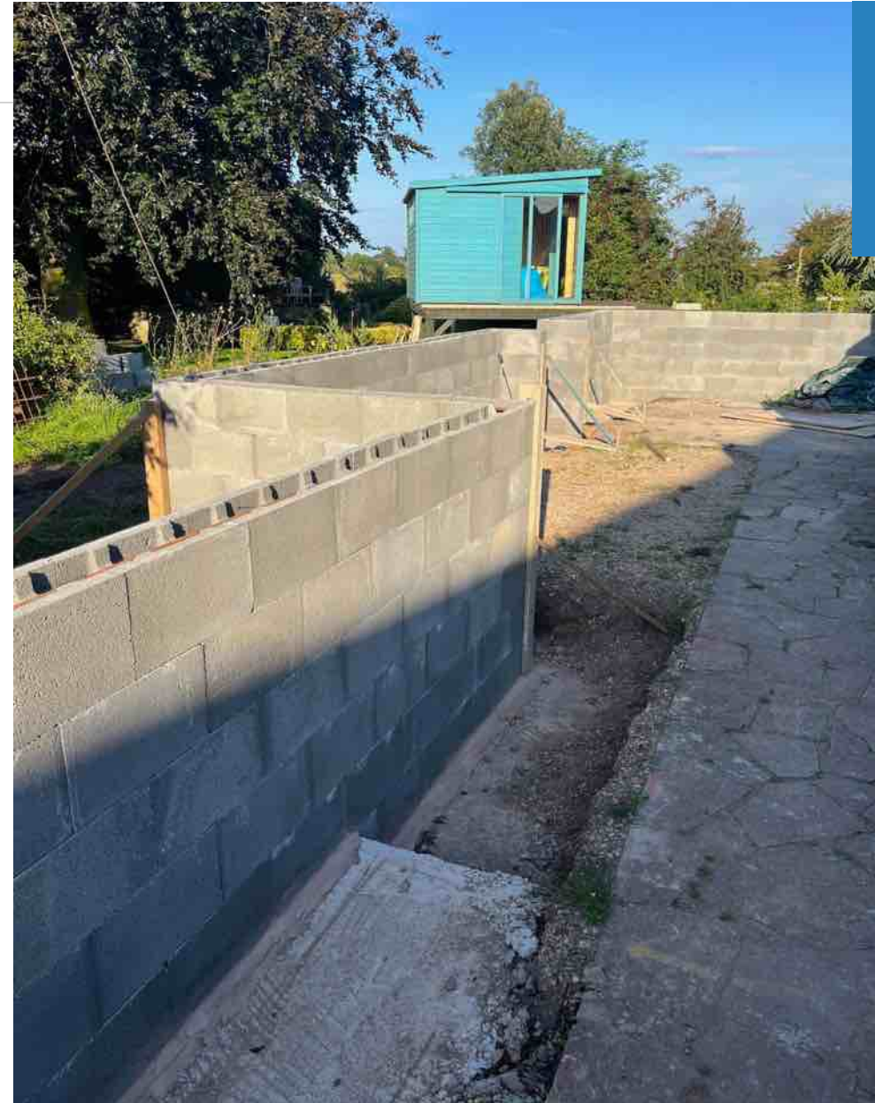
Where the wall joined the garage block it was cut into the existing brickwork to ensure stability and a strong watertight seal.
