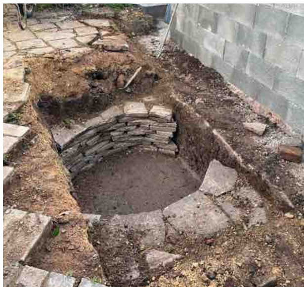
The paving slab 'well'
