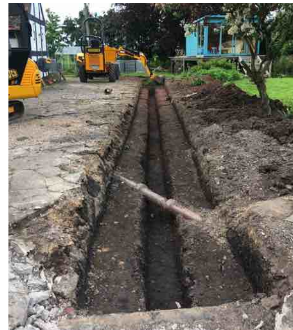
Centre trench excavated
