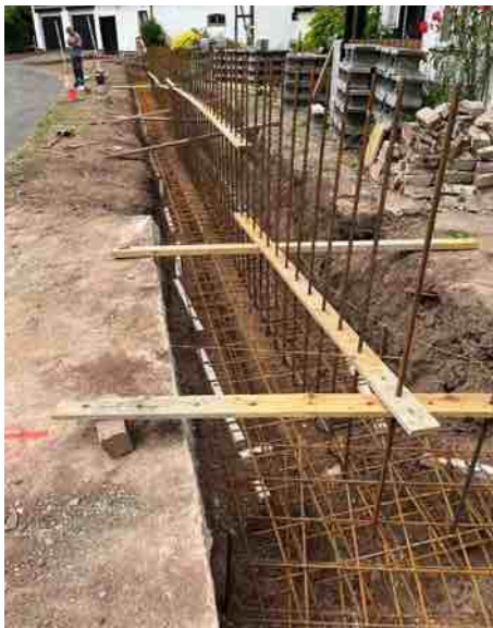
We used timbers with holes drilled, to ensure the bars remained correctly spaced and vertical during the pour
