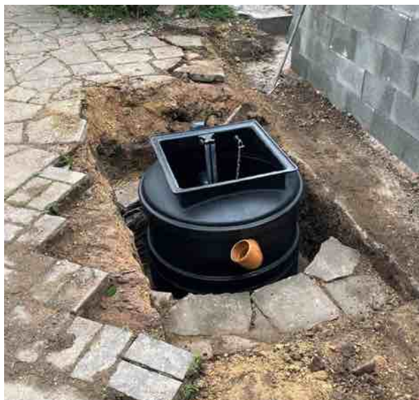
Sump in place ready for concrete
