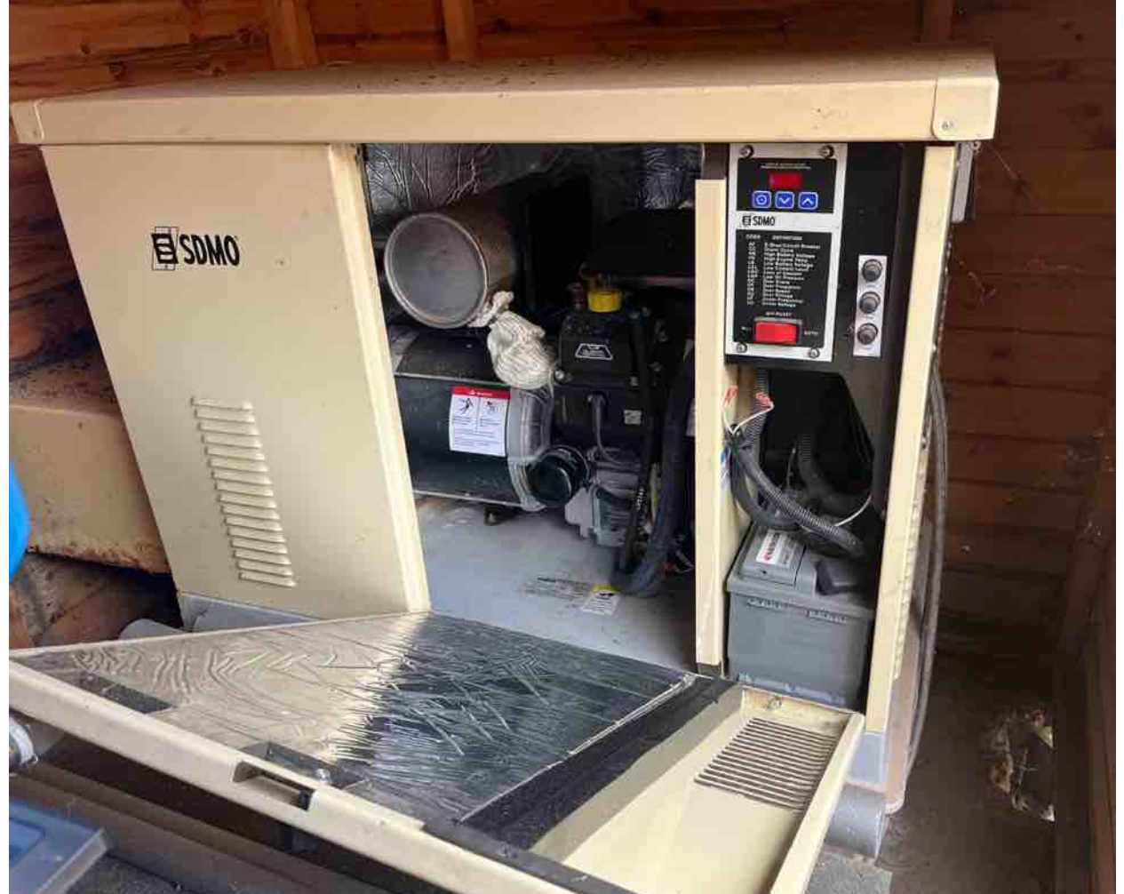
LPG Backup generator, strong enough to run the pumps during a power cut.
